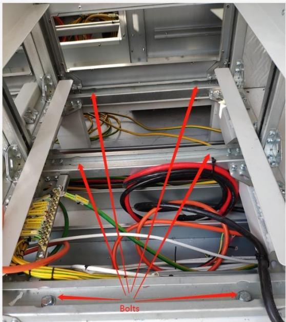
The positions of bolts are shown in the picture, which are anchored into ground. The
